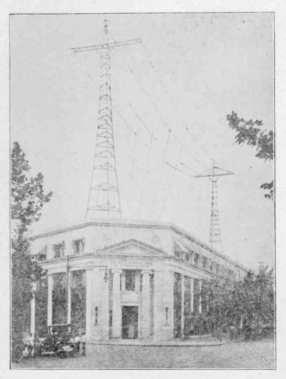
Fig. 1. Elaborate Aerial System at WRC
